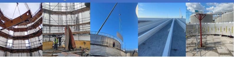
UnitBirwelco's Unit Engineers & Constructors Storage Tank Division has been appointed as the Principal Contractor for an ongoing storage tank replacement project in East Yorkshire, UK. The project involves the replacement of two existing carbon steel storage tanks—a 3000T tank (21.5m diameter x 10m high) and a 500T tank (7.5m diameter x 13m high)—with new tanks of identical size, constructed from 304L stainless steel. The project is scheduled for completion in May 2025.
